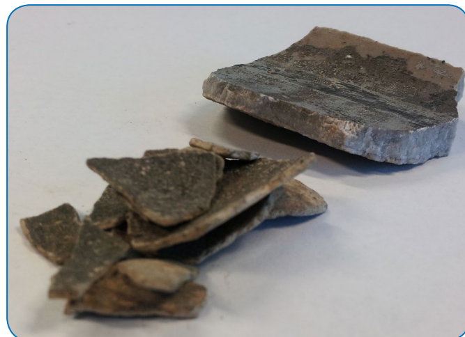
Figure 1: Two scale deposits that were mechanically removed from pipe segments for analysis and testing.
